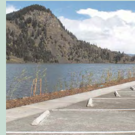
Pervious concrete filters water through a permeable subbase and the soil below, preventing contaminated water from entering waterways or stormwater management systems.
