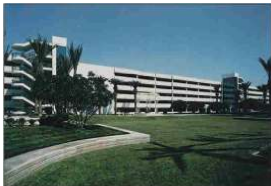
The use of light-colored concrete and good landscaping are a winning combination for the reduction of heat-island effects.
