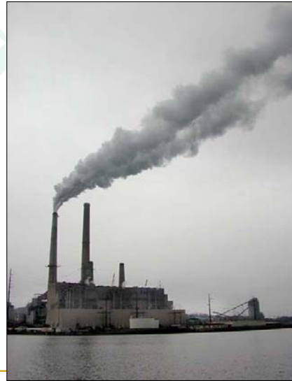
Coal fired electric power plant
