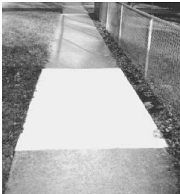
Figure 2. New PCC section in weathered PCC sidewalk.
