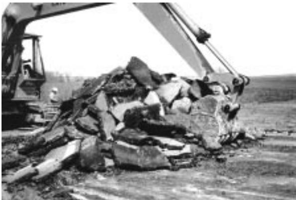
**Figure 13. Removal of ACC pavement for recycling. (S-38441)**
