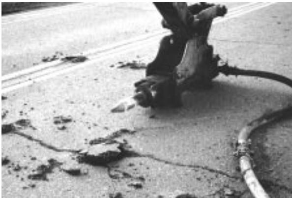
**Figure 12. Loosening of ACC pavement before removal. (S-39363)**
