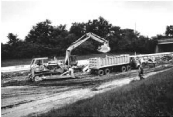
Figure 10. Removal of PCC for recycling. (S-42534)
