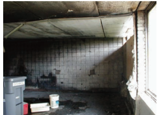
Source: Northeast Fire Safety Construction Advisory Council Fire resistant non-combustible materials contain fires minimizing fire and smoke damage. This damage resistance allows portions of the buildings to simply be cleaned, painted and reoccupied rather than completely re-constructed.
