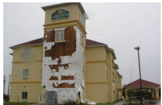
Source – Institute for Business & Home Safety
