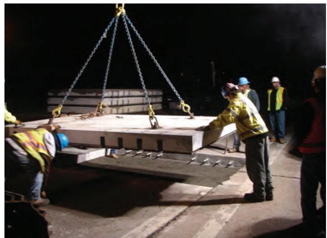
Figure 3.3 Precast pavement being installed (photo courtesy of Shiraz Tayabji, FHWA)
