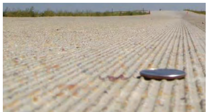
Figure 5.11 Diamond-ground texture (Rasmussen et al. 2008)
