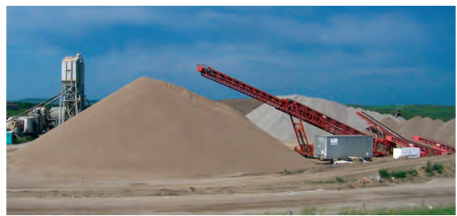
Figure 5.3 Stockpiling aggregate with a radial stacker (photo courtesy of Gary Fick, Trinity Construction Management, Inc.)
