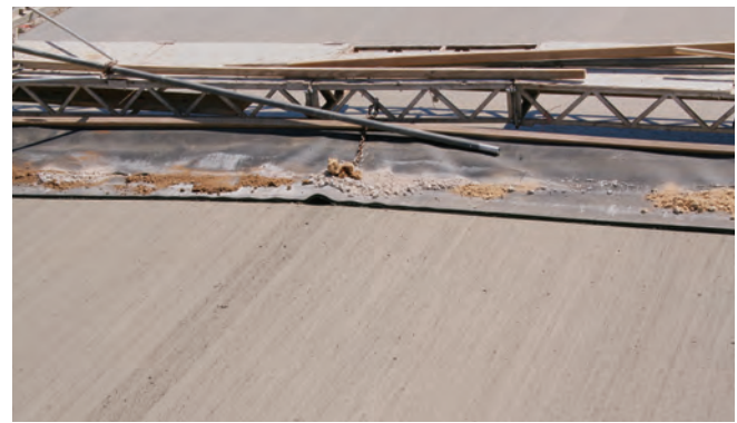
Figure 5.10 Artificial turf drag texture (photo courtesy of Gary Fick, Trinity Construction Management, Inc.)
