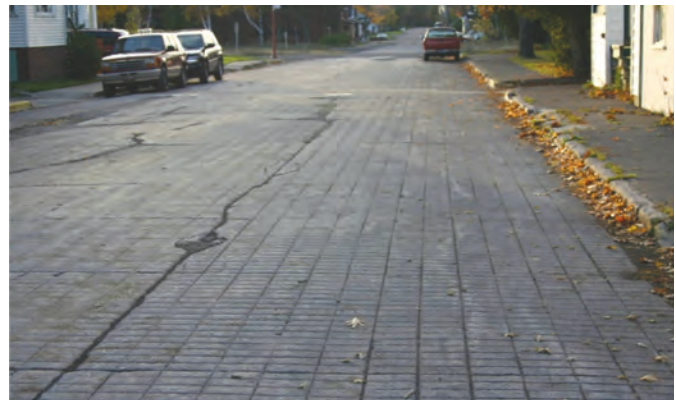
Figure 9.4 Blome Granitoid concrete pavement constructed in 1906 in Calumet, Michigan; the brick pattern was stamped into the surface to keep horses from slipping (photo courtesy of Tom Van Dam, CTLGroup)
