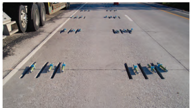
Figure 7.7 Dowel bars on chairs with end caps and compressible inserts in place ready to be inserted into prepared slots (IGGA 2010)
