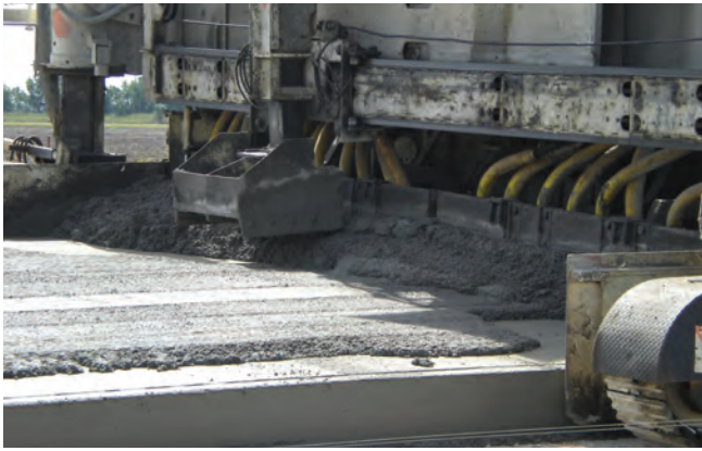
Figure 5.12 Top lift being placed on the bottom lift (photo courtesy of Gary Fick, Trinity Construction Management, Inc.)
