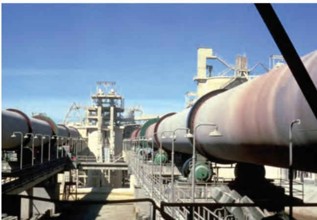
Figure 4.1 A cement kiln (photo courtesy of PCA)
