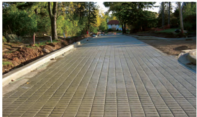
Figure 9.5 Modern Blome Granitoid concrete pavement (photo courtesy of Tom Van Dam, CTLGroup)
