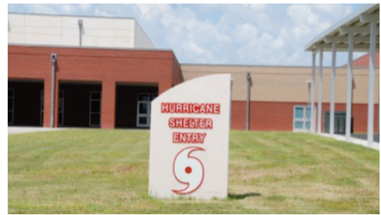
Source: Federal Emergency Management Agency, photograph taken by Tim Burkitt of FEMA.
