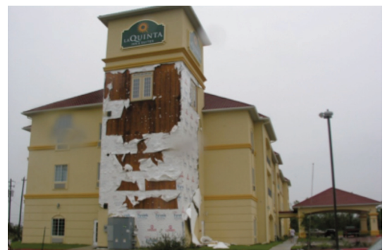
Source - Institute for Business & Home Safety
