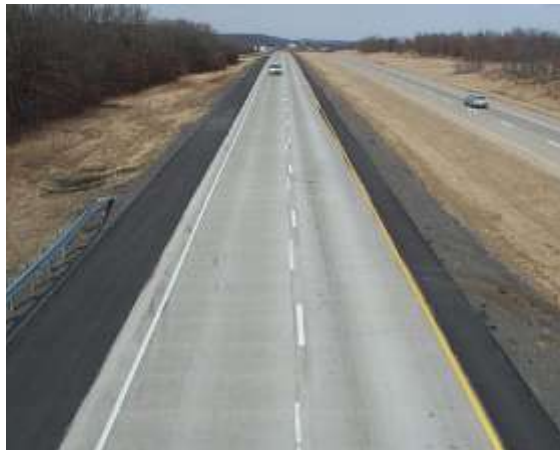
Whitetopping is gaining in popularity in fixing deteriorating hot-mix asphalt pavements and includes the benefit of having a higher albedo, better performance and increased durability over asphalt.
