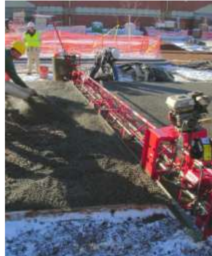
Pervious concrete paving example – placing pervious screed.
