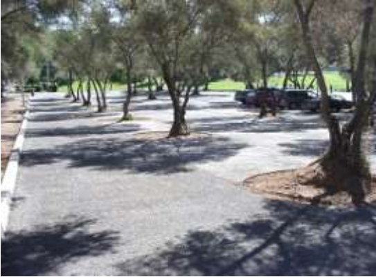
Pervious pavements allow for groundwater recharging while also assisting with water pollution removal.
