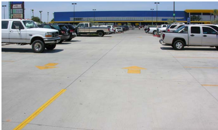
Figure 6 Portland cement concrete parking lot in Tempe, Arizona. Photo courtesy of National Center of Excellence, Arizona State University.
