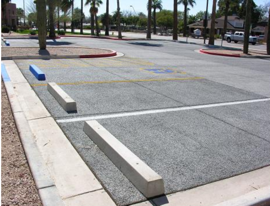
Figure 21 Pervious concrete parking lot located at the J. Russell and Bonita Nelson Fine Arts Center on the main campus of Arizona State University in Tempe, Arizona.
