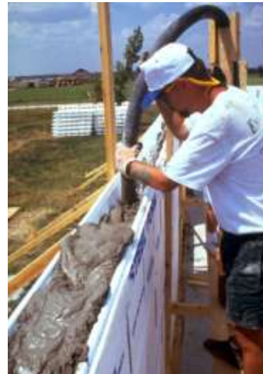
ICF buildings have long been known to be particularly energy efficient.
