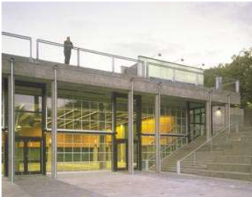
Concrete offers several opportunities for building projects to gain LEED points.
