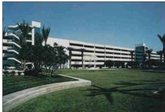
The use of light-colored concrete and good landscaping are a winning combination for the reduction of heat-island effects.
