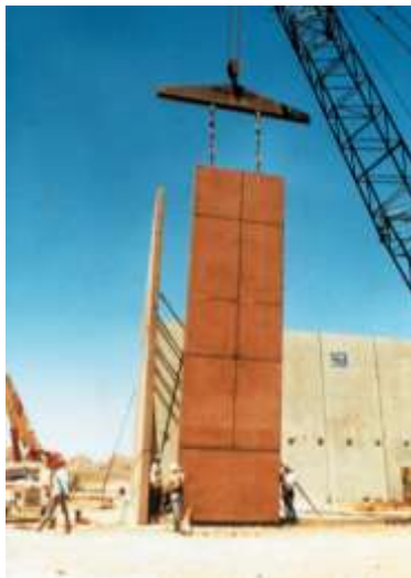
Tilt-up construction is often used to save on energy costs.
